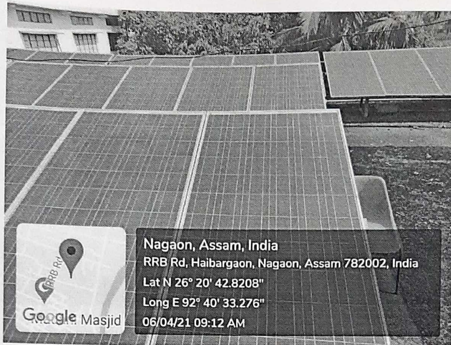
Solar Panel Installed at rooftop
